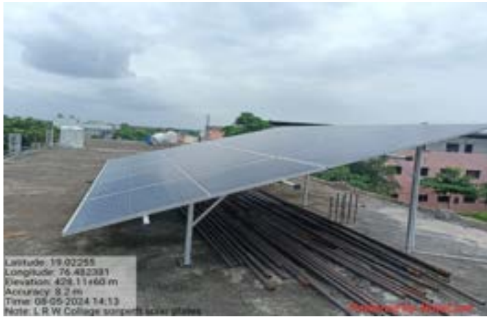
Solar Panels are installed in college
