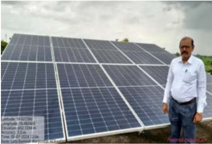
Solar Panels are installed in college
