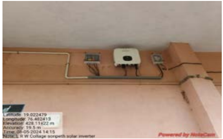
Wheeling to the Grid
